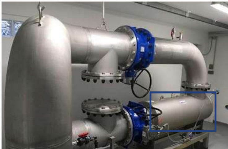
Connecting UV reactors to the network.
